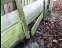
The heavy-duty gravel board of the fence (bottom left) has been displaced by crown growth in the adjacent property.
