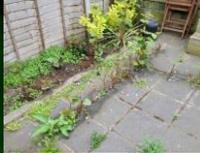
Patios, block paving and concrete are all vulnerable to Japanese knotweed, which will exploit cracks, joints and weak areas. The damage, if left untreated, simply worsens over time as the knotweed rhizome and/or crown grows and expands.
