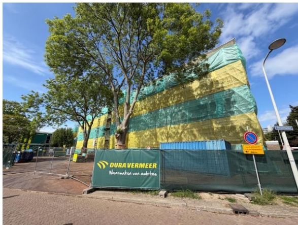
Mariahoeve renovation site, The Hague (contractor: Dura Vermeer)
