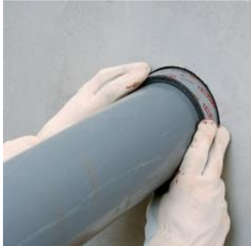
CFS-W EL Pipe Wrap Up to 240mins fire rating 50mm up to 160mm
