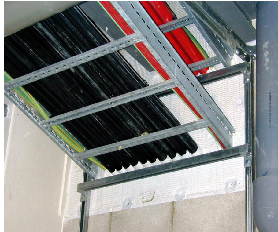
CP 670 Coated Board Up to 240mins fire rating
