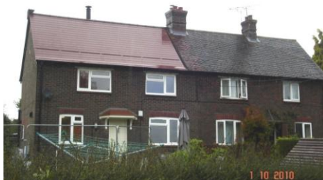
Roof based energy collector
