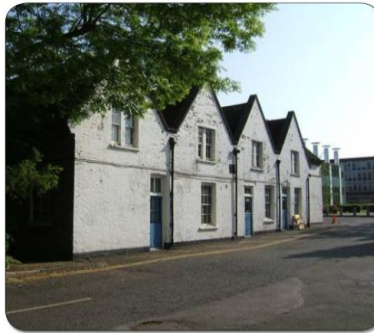
BRE's flagship refurbishment project
