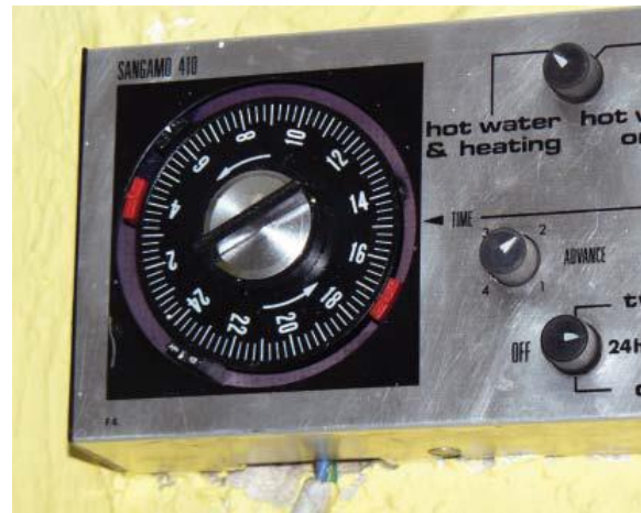
Cable sheath not within metal enclosure
