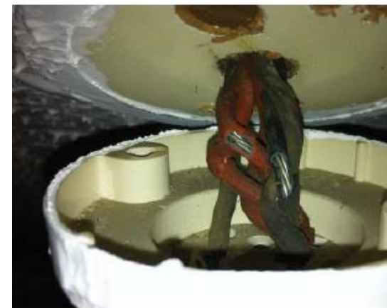
Crumbling vulcanised rubber insulation
