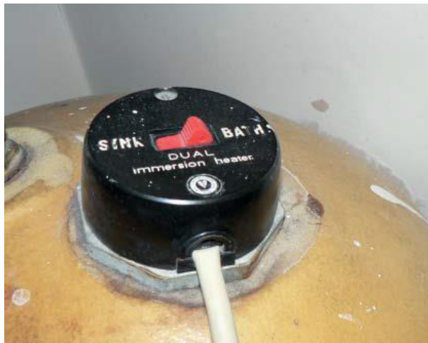
Old Immersion heater without thermal cut-out
