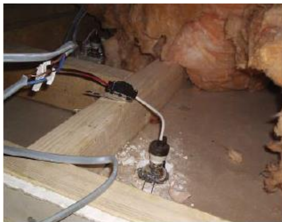
Unsatisfactory electrical connections
