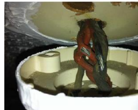
Crumbling vulcanised rubber insulation
