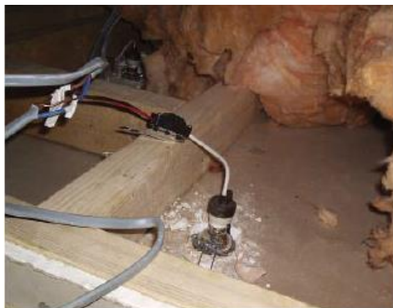
Unsatisfactory electrical connections
