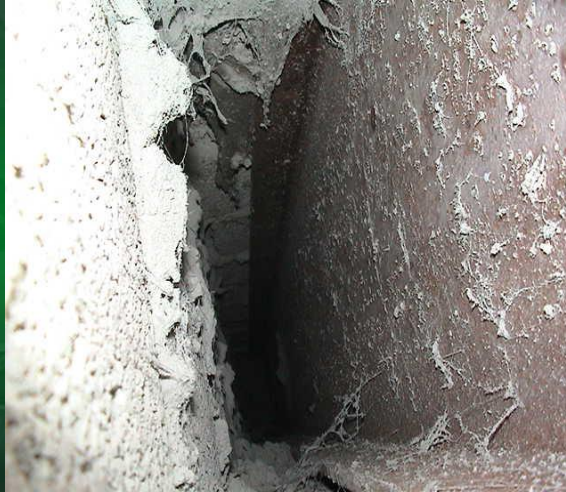
Asbestos Debris Hidden Within Ducting (after previous removal?)
