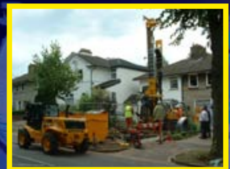
Ground Source Heat Pump hole drilled 65 metres into the ground.
