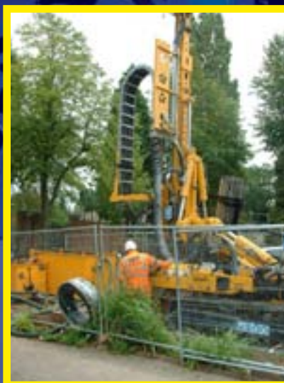
Ground Source Heat Pump hole drilled 65 metres into the ground.
