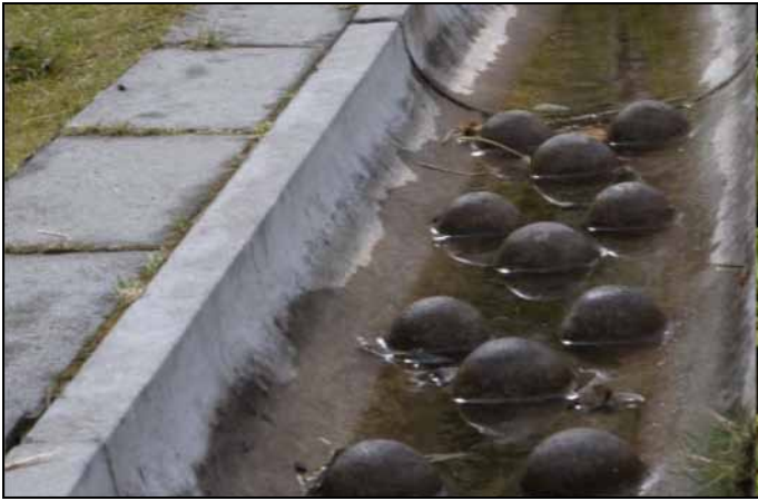
Knobbles cause turbulence which stops clogging by leaves
