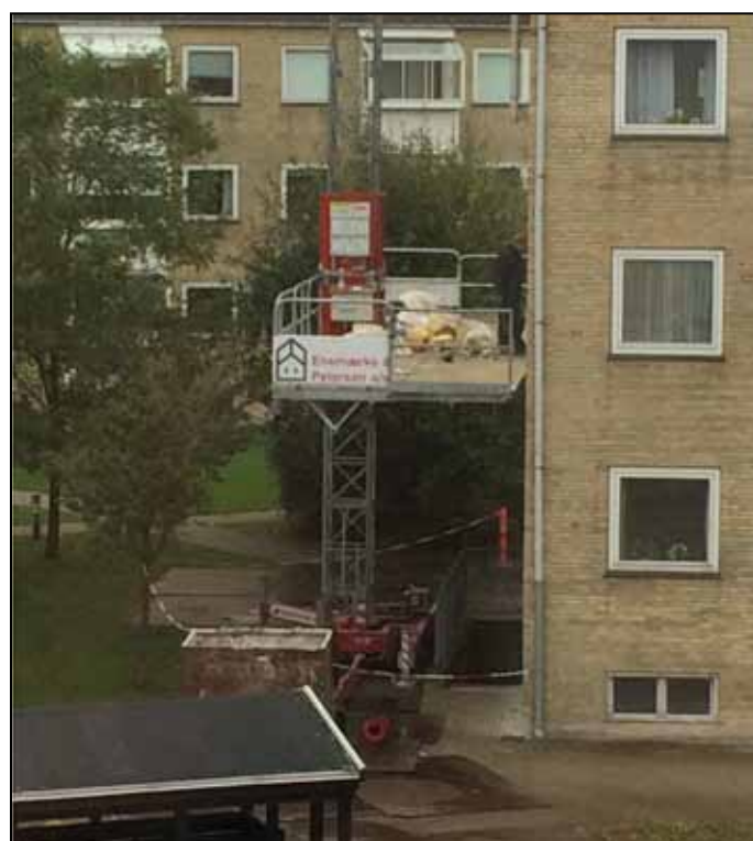
Repointing, and window & lintel replacements
