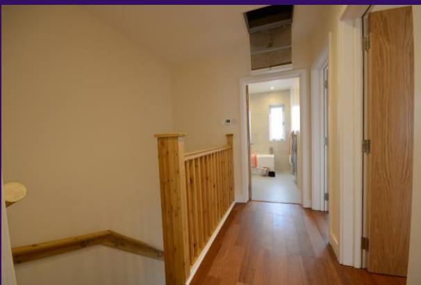
Airtightness test with Open Roof Hatch 2.9\text{m}^3/\text{hr}/\text{m}^2@50\text{Pa}
