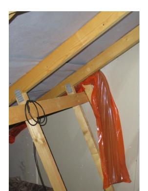
Check for fire stopping tightly fitted to head of spandrel. NOT like this!
